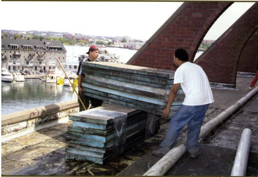
Figure 5 – The extruded polystyrene was re-used at other locations.
