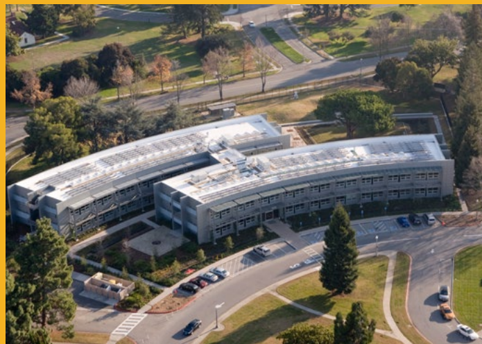
NASA's Sustainability Base in Moffett Field, California, is considered the federal government's "greenest" building and features a Sika Sarnafil EnergySmart Roof®.
