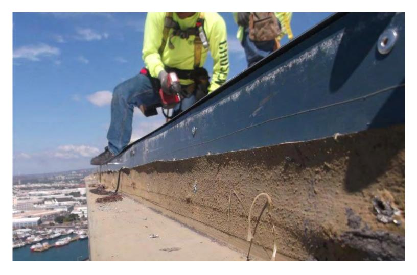
CRW's first task was to remove the five existing arched panels and create a customized fabricated curtain wall cap flashing that encapsulated the head of the curtain wall system for a watertight seal. "The clad flashing was a critical detail to prevent future leakage into the wall," Garlin stated. "I like that Sika offers stainless steel with PVC cladding, which is a better option for salt air exposures."
