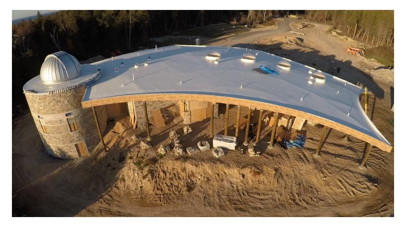
Bloxsom Roofing. "Everything on this project had a radius, thus requiring the 6-8 relief cut and stripping. There were also four large skylights, a 10-foot diameter chimney, and a dozen or more light pipes, all giving our roof detail specialist a work-out."
