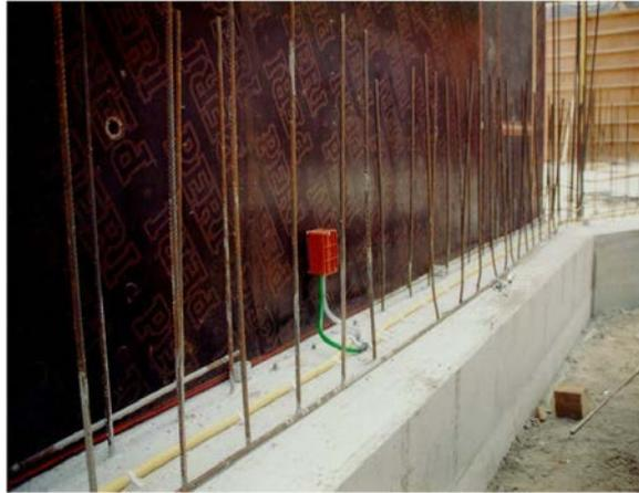
Figure 2: vent ends entering junction box
