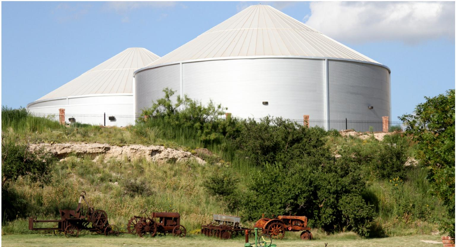
remarked. “All the pieces of the roofing membrane had to be measured and cut into pie-shaped pieces to wrap around the cone.”
