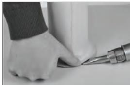
5. Slide the flashing, scalloped-end down, back onto the vent. Hot-air weld the scalloped flange to the base plate. Hot-air weld the base plate to the field sheet. Trim the top of the flashing even with the top of the stack. Finish with clamping ring and sealant 8" (20.3 cm) above the field sheet.
