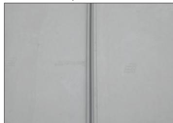
Fig. 1.2 Positioning Décor on membrane overlap
