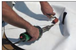
6. Weld the top lap. The entire lap is fully welded from the center of the target patch to the outside.
