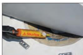
8. Apply one full tube of Sikaflex-1A or approved sealant per TB 23-01 to the drain bowl flange.
