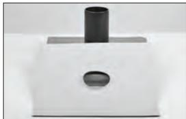
1. Cut field sheet tight to the vent stack. From membrane, cut a base plate large enough to provide a 5" (12.7 cm) flange.
