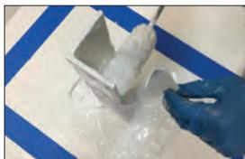
8. Embed the pre-cut vertical Liquid Flashing Fleece into the wet Liquid Flashing. Use the roller or brush to eliminate wrinkles and air bubbles while completely saturating the Liquid Flashing Fleece. Apply additional catalyzed Liquid Flashing at the 2" (51 mm) overlap between the vertical Liquid Flashing Fleece layers.
