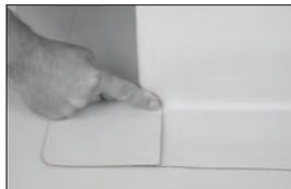
8. Cut oversize piece from membrane; cut rounded corners. Enlarge one of the corners by heating and flanging it so that it will extend over the base of the outside corner (this step may be replaced by using a Sarnacorner).
