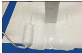
9. Apply 55 mils (1.4 mm) of catalyzed Liquid Flashing onto the roof membrane extending slightly onto the painters tape, also coat the 2" (51 mm) fingers from the vertical Liquid Flashing Fleece.
