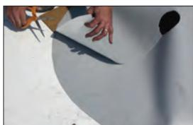
4. Flip the target patch over and trim off excess membrane leaving 2" - 3" (51 mm - 76 mm), round the top layer and cut the bottom layer
