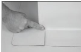
9. Trim the patch so that it extends neatly past the outside corner and overlaps the flashing a minimum of 3/4" (19 mm) in all directions (this step is not needed if Sarnacorner is being used).
