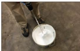
5. Thoroughly stir the entire container of Liquid Flashing with a slow-speed (200 to 400 rpm) mechanical mixer (electric drill with a mixing blade) for two minutes.
