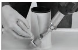
7. After welds are thoroughly cooled, check all welds with a rounded screwdriver blade. Reweld any inconsistencies.
