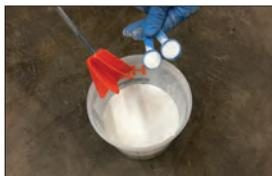
6. Pour 1 liter of Liquid Flashing into a clean plastic container. Add Liquid Flashing Catalyst to Liquid Flashing SW at rates depending on ambient temperature (see Mixing Rates table). Mix using a slow-speed mechanical mixer with a separate mixing paddle for two minutes. Once mixed, the pot life is approximately 10 - 15 minutes depending on the ambient temperature.
