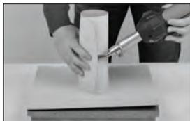
3. Install a spacing strip slightly longer than the height of the vent stack loosely to the vent stack. Wrap the vent stack with flashing membrane, allowing for an approximately 1" (25 mm) overlap, and hot-air weld the overlap
