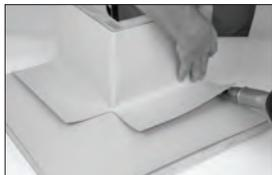
5. Set flashing in place. Overlap previous flashing sheet by 4" (10.2 cm). Keep top edge of flashing level with termination line. Do not allow flashing membrane to bridge at base of curb or wall.
