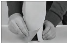
4. Slide out the spacing strip and remove the now tubular flashing. Flange the bottom of the flashing by applying moderate heat and stretching the membrane, creating a scalloped effect.
