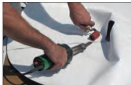
6. Weld the top lap. The entire lap is fully welded from the center of the target patch to the outside.
