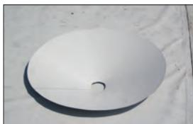
3. Center the target patch over the drain pipe and allow it to conform to the sump. Lightly tack the lap to hold the target in the desired shape.
