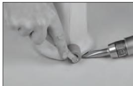
6. Install a separate piece of membrane flashing so that it extends into the stack (dark side of membrane should be facing out) a minimum of 4" (10.2 cm), tight to the inside diameter of the stack and extending a minimum of 1" (25 mm) above the stack. Bend the protruding part of the internal flashing so that it is tight to the external stack flashing. Hot-air weld the overlap.
