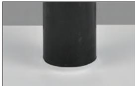
2. Cut a hole in the center of the baseplate membrane that is 1/2" (13 mm) smaller than outside diameter of the stack. Stretch the base plate down over the stack until it is flat on the field sheet, except where it will neck up the base of the stack.
