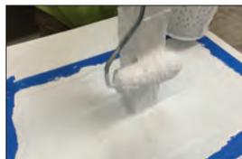
11. Apply 25 mils (0.6 mm) of catalyzed Liquid Flashing over the entire exposed vertical and horizontal flashing fleece terminating at the finished flashing height on the vertical and onto the painters tape on the roof. Make sure the fleece is fully saturated without any dry spots.
