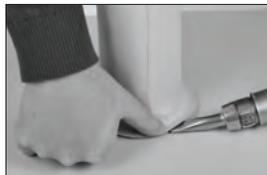
5. Slide the flashing, scalloped-end down, back onto the vent. Hot-air weld the scalloped flange to the base plate. Hot-air weld the base plate to the field sheet. Trim the top of the flashing even with the top of the stack. Finish with clamping ring and sealant 8" (20.3 cm) above the field sheet.
