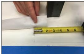
penetration allowing for a 2" (51 mm) overlap with adjoining pieces.
