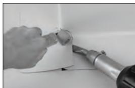
9. Trim the patch so that it extends neatly past the outside corner and overlaps the flashing a minimum of 3/4" (19 mm) in all directions (this step is not needed if Sarnacorner is being used).
