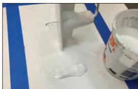
7. Using a small ½" (13 mm) nap roller with rounded edges or 2" (51 mm) disposable paint brush apply 55 mils (1.4 mm) of catalyzed Liquid Flashing onto the penetration up to the finished flashing height and 2" (51 mm) onto the roof membrane.
