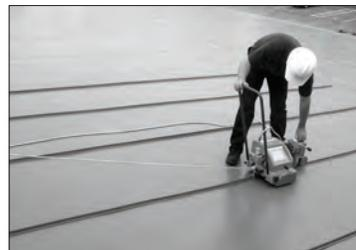
Fig. 1.5 Safety rope securely attached to the automatic welder
