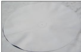
2. Cut a round target patch. The target patch must be large enough so when installed there will be a minimum of 2" - 3" (51 mm - 76 mm) coverage past the fasteners / plates and relief cuts. Cut the target from one edge to the center as shown. Cut the hole in the target patch slightly larger than the diameter of the drain pipe.
