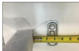
1. Horizontal flashing fleece pieces must extend a minimum of 4" (10.2 cm) beyond the leading edge of the penetration.
