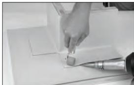
6. Cut the flashing square at the base of the curb or wall and wrap it around the corner. Rub in flashings with a hand roller to ensure full adhesion.
