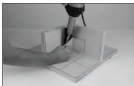
2. Coat the curb or wall with Sarnacol 2170 or 2170 VC adhesive. Allow adhesive to dry.
