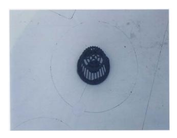
**Custom Insert** – The above detail should work with most drains. For extreme situations, with even steeper sumps or for no sump drains, (such as found near a corner at a parapet wall) a custom prefabricated, PVC drain insert can be purchased through Sika-Roofing.
