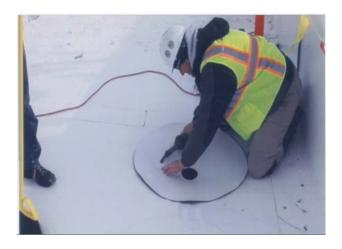
**Step 3-** Center the target patch over the drain pipe and allow it to conform to the sump. Lightly tack the lap to hold the target in the desired shape.
