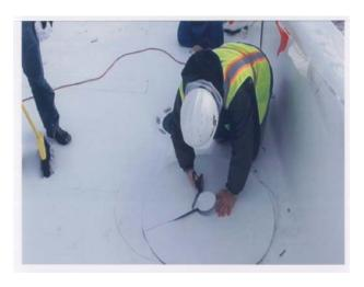
Step 2 –Cut a round target patch. The target patch must be large enough so when installed there will be a minimum of 2"-3" coverage past the fasteners / plates and relief cuts. Cut the target from one edge to the center as shown. Cut the hole in the target patch slightly larger than the diameter of the drain pipe.
