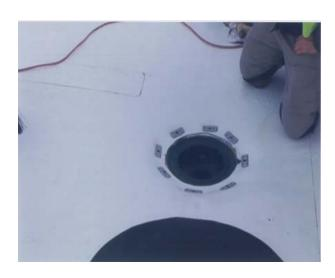
Step 1. This photo shows a condition where the insulation has been shaved with a saw. Position the field membrane and trim close to the drain bowl. Membrane is to lay flat, pie shape relief cuts may be required. Install the specified fasteners and plates to secure the field membrane. Installing the fasteners in the sump rather than on the flat area will make it easier to transition the target patch without wrinkling.
