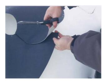
**Step 4-** Flip the target patch over and trim off excess membrane leaving 2"-3", round the top layer and cut the bottom layer at a 45° angle.
