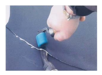
Step 5- Pre-weld and finish weld the back side lap completely. This step is critical to prevent water migration into the roofing system in case of a drain back up. Chafer finish weld using the hot air gun, creating a smoothness to the weld.
