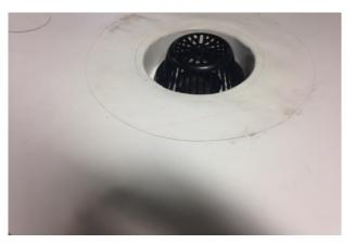
When using a pre-fabricated drain insert, a drain basket must be used which is higher than the roof plane. This will help prevent clogging. Please contact Sika-Roofing Technical Department for more information on measuring and ordering custom drain inserts.
