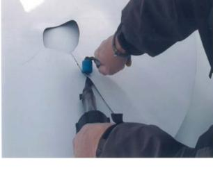
**Step 7-** Place the bolts to hold the target in place. Do not place welded seam on a bolt. When possible, position seam away from direct water flow (high side) of drain.
