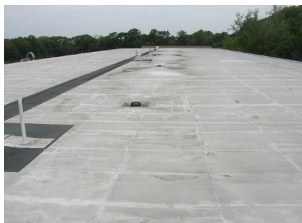
Photo 2: Open roof with long, black walk pads
