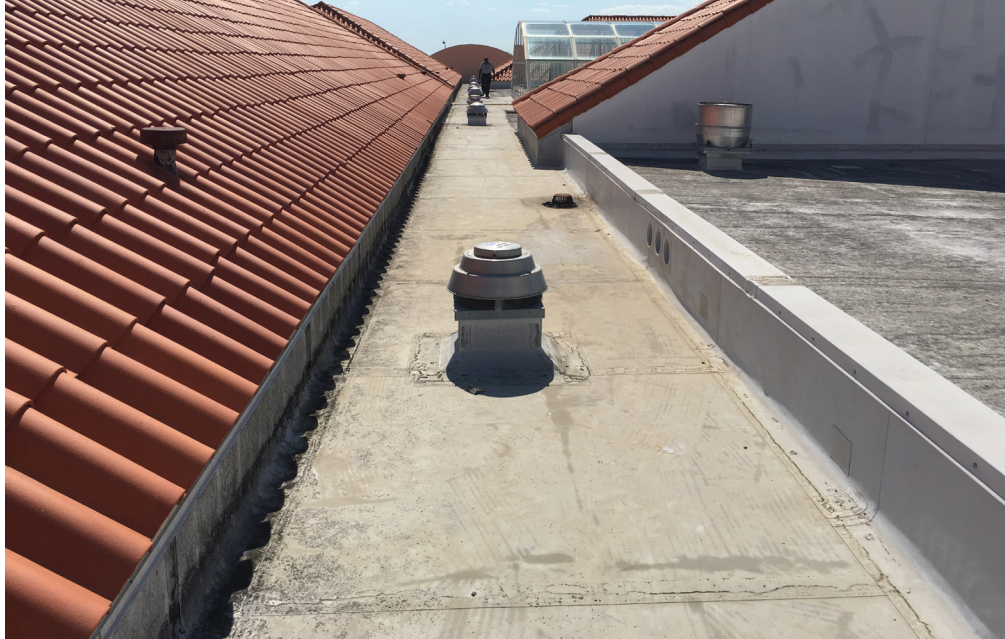
Photo 1: Miami roof with clay tile
