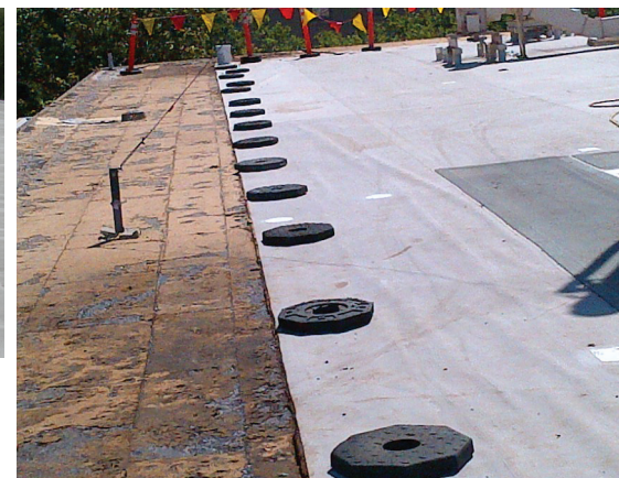
Photo 3: Perimeter tear-off with perlite
