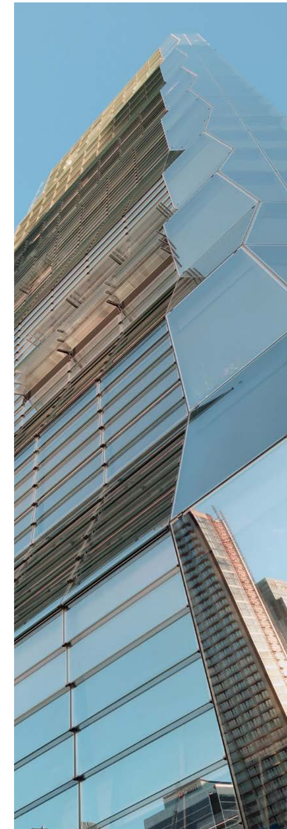
Dollar Bay, London, 2017 Architects SimpsonHaugh; Facade and balustrades Focchi Spa (IT)
