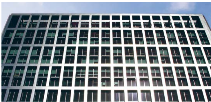
5 Aldermanbury Square, London, 2005 Architects Eric Parry Architects; Facade Lindner-Schmidlin UK
