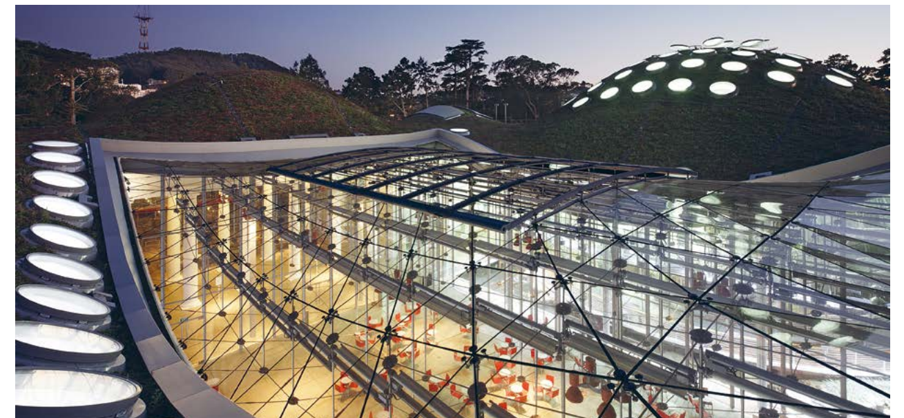
California Academy of Science, Exhibition and Research Center, 2008 Architects Renzo Piano Building Workshop, Stantec Architecture; Facade Josef Gartner (DE)
