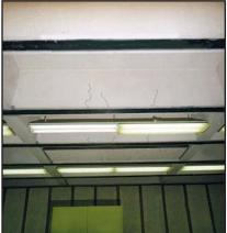
The structural evaluation revealed that the majority of the cracks in the visible bottom part of the joists were flexural cracks anticipated in the original structural design.
