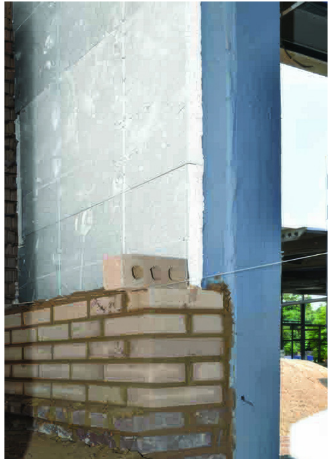
Finestop air/water-resistive barriers can provide a continuous air and water-resistive barrier behind multiple claddings for uninterrupted air and moisture protection
