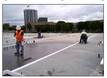
**Sikadur® 32, Hi-mod –** a multi-purpose, 2-component, 100% solids, moisture-tolerant structural epoxy adhesive. It conforms to the current ASTM C-881, Types I, II, and V, Grade-2, Class C and AASHTO M-235 specifications. **SikaLevel® 315 –** a multi-purpose, 2-component, 100% solids, moisture-tolerant structural epoxy adhesive. It conforms to the current ASTM C-881, Types I, II, and V, Grade-2, Class C and AASHTO M-235 specifications.
