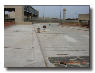
The specification called for a new long lasting epoxy broadcast system that would provide good skid resistance and make the elevated deck waterproof. The total area that needed to be repaired and recoated included:
