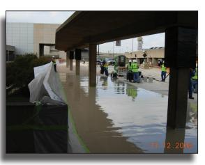
The pigments were matched and samples were provided to the GC and Owner in less than a week, with the help of representatives from Sika's Industrial Flooring Business Unit. The epoxy was pigmented on site to match both the dark brown and light tan aggregates. This combination of pigmented epoxy and the colored aggregate will help to minimize the natural discoloration typically seen in epoxy over time.
