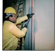
Finally, the surface of the tank walls was protected using Sikagard® 62, a high-build epoxy protective coating. All repairs were made using NSF/ANSI standard 61 approved products for drinking water contact.
