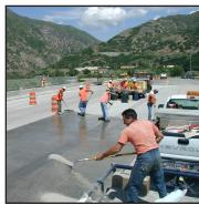
When material levels, broadcast aggregate slowly, allowing it to settle into epoxy.
