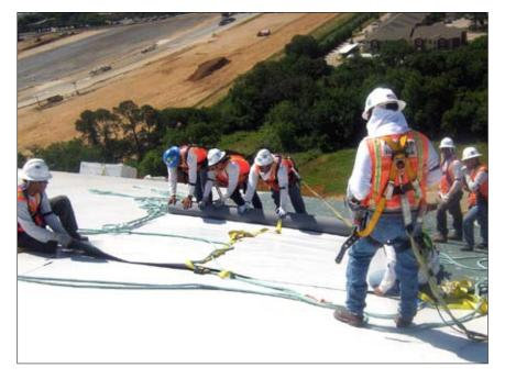
was installed, along with insulation and roof board, over concrete, metal and acoustical decks, and seams were hot-air welded to ensure a watertight seal.
