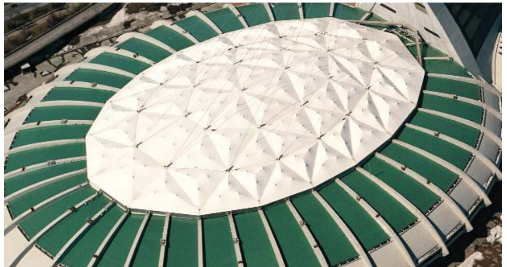
G410 membrane installed in between roof's curves
