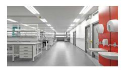
Resilient sheet goods minimize the seams as compared with tiles and are manufactured with a protective coating to minimize maintenance costs. Welded seams are potential areas for system failure, especially in wet areas. Expected life will be limited in the area receiving the most aggressive wear pattern. Replacement may be more expensive than initial installation due to removal and surface preparation requirements.
