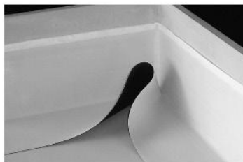
Internal corners, fabric edge above
