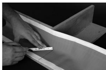
Mark a 45° angle to the corner on the Sika® Dilatec® E tape .
