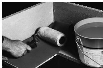
Internal corners, fabric edge below
