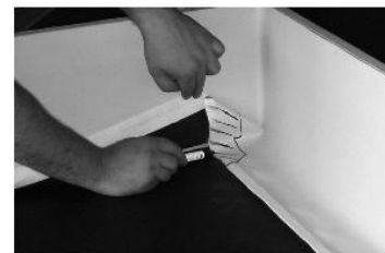
Internal corners, fabric edge below
