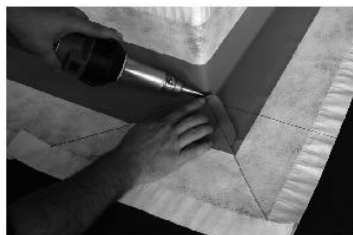
Fit the tape section, start welding at corner.
