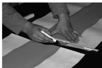
B type butt joints
