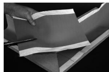
Trim surplus material from the Sika® Dilatec® E tape and cut off the fabric edge on one side only.
