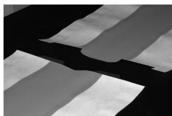
Sealing strip butt joints
