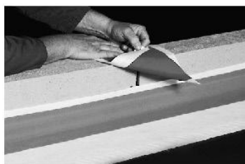
Sika® Dilatec® E in the joint area.
