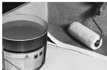
Internal corners, fabric edge above
