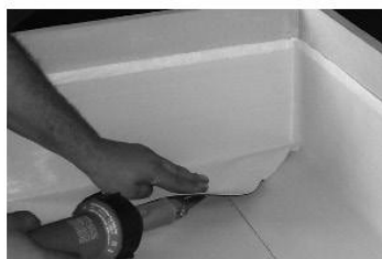
Internal corners, fabric edge above
