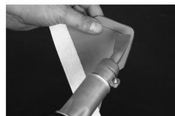
Cut the tape sections, heat the corner area and shape.
