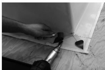
Cut the sealing tape for the butt joint area.
