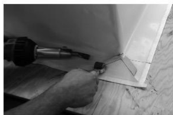
Weld overlaps in the movement area.
