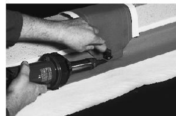
Weld the T-junction lap
