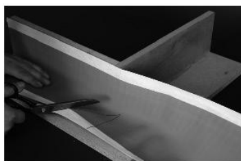
Cut tape and fit around the external corner without any creases. The movement area can be held with Sika® Contact Adhesive C-733 as an assembly aid.
