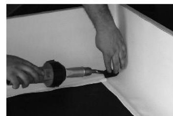
Internal corners, fabric edge below
