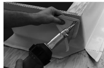
Cut the tape section, heat the corner area and shape.
