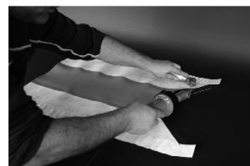
Cut the edge tape for the butt joint area.
