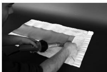
Finish welding the movement area.
