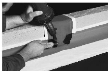
Sealing strip T-junction
