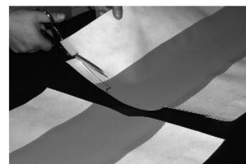
Cut the butt joints
