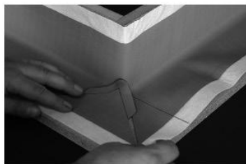
Fit the tape section, start welding at the corner.
