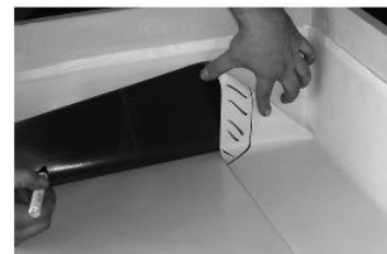
Internal corner, fabric edge above
