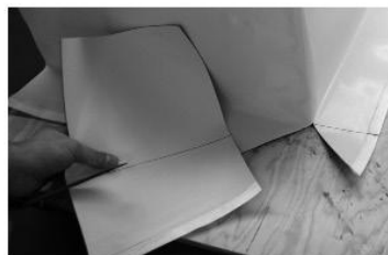
Cut surplus material from the Sika® Dilatec® ER tape to size.
