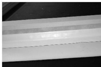
Sika® Dilatec® E epoxy-bonded installation
