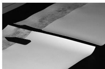
Cut the sealing strip tape joint
