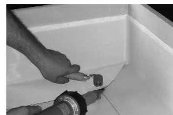
Internal corners, fabric edge above
