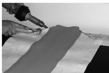
Hold the T-junction together
