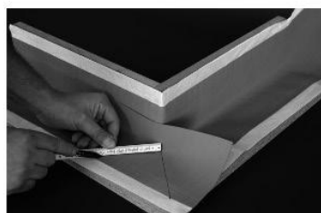
Mark 3 points on tape section.
