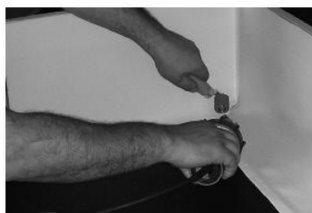
Fabric edged internal corner welding
