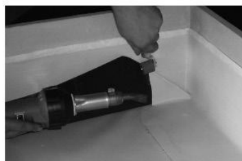
Internal corners, fabric edge above
