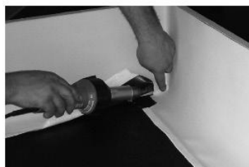
Internal corners, fabric edge below
