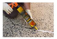
Clean up all tools, spills, and excess material with clean rags after use. If necessary, use a paint thinner or other approved solvent, such as acetone, following the solvent manufacturer's precautions.
