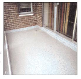
**Protection -** All balcony waterproofing was carried out using Sikadur 22 Lo-Mod, a two-component, solvent free epoxy resin, which when broadcast with a blended, colored aggregate, provides an attractive, highly durable, slip resistant, waterproof wearing course.
