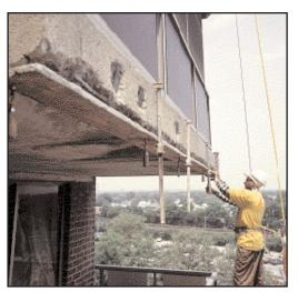
Rochdale Village, home to over 20,000 people, is comprised of twenty 14-story buildings constructed in the late 1960's. A combination of carbonation and inadequate cover to the reinforced concrete balconies had caused extensive cracking and spalling of concrete cover, resulting in loss of concrete and a clear potential safety issue.
