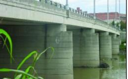
sidewalk. The storm water picked up all deleterious materials, especially de-icing salts, and deposited them onto the exposed side of the fascia box beams.
