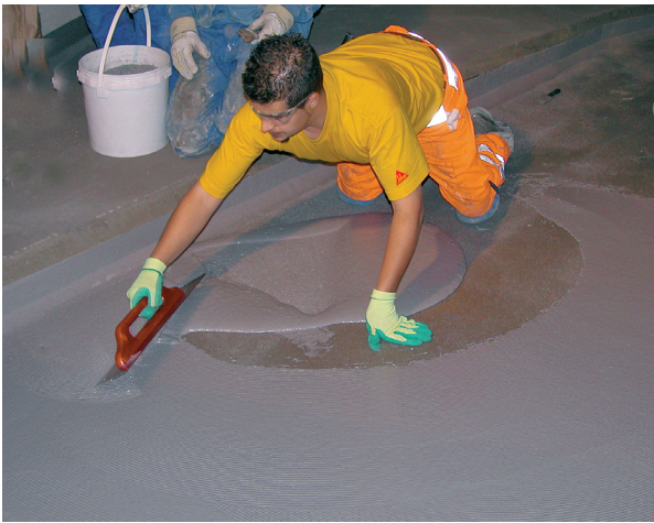
Sikafloor® Marine primary deck covering mortars are easy to apply with a steel tube or a straight edge.
