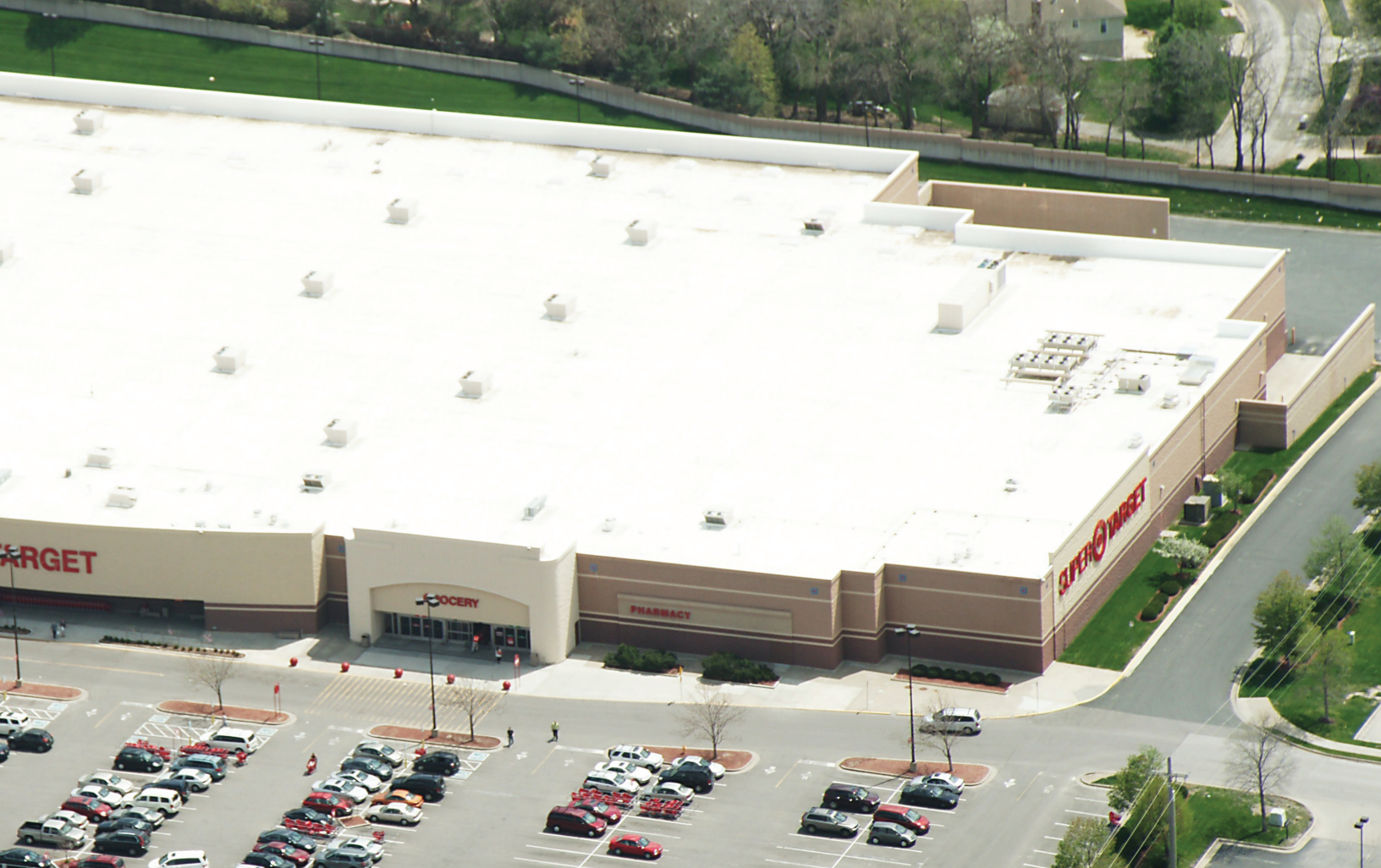
▲ In 2012, a new, long-lasting Sika roof was installed on the SuperTarget retail store in Olathe, KS in a reflective, energy-efficient white color. The old vinyl roof totaling 175,000 sq. ft. was removed and shipped to Sika for recycling into new roofing product.
