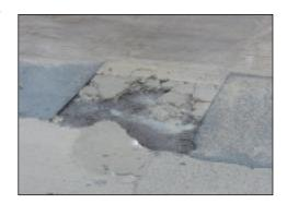
Spalling of concrete on the bridge deck led to an investigative analysis. The analysis indicated that the quality of the concrete cover was poor and in many areas insufficient in depth. The bridge is also exposed to an aggressive envi-
