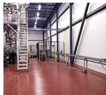
Wells Restoration used polyurethane cement technology because it is less sensitive to temperature changes. "This floor was going into an area that was basically a big cooler with a temperature of 35°F, so I knew the urethane cement would meet these environmental conditions the best." Wells said.
