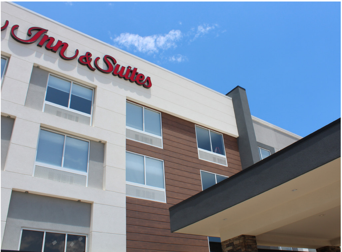
Senergy Channeled Adhesive CI Design, incorporating Sika's Wood Grain Effects, can produce an energy efficient building with endless design possibilities.
