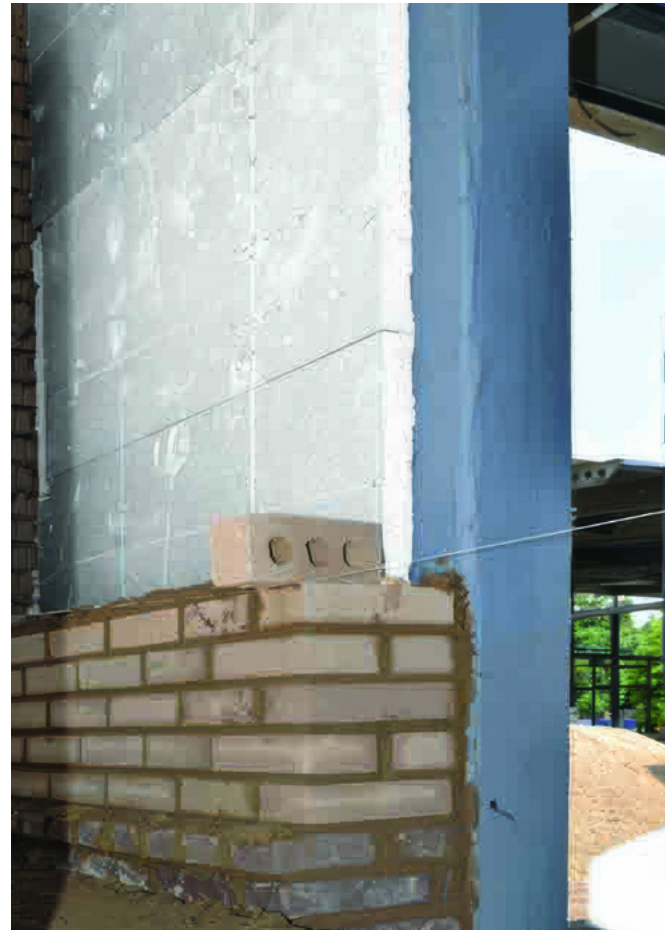
Senershield air/water-resistive barriers can provide a continuous air and water-resistive barrier behind multiple claddings for uninterrupted air and moisture protection
