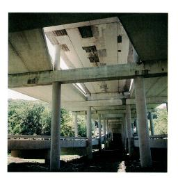
Reinforced concrete access ramps, approximately 20 years old, were suffering from water and deicing salt penetration causing corrosion of reinforcing steel. The chlorides had penetrated by diffusion to reach the steel and caused spalling and delamination in the topping slab. In other areas, cracks allowed the chlorides through the slab leading to corrosion of the steel closest to the underside of the ramps, as well as in the beams and columns.
