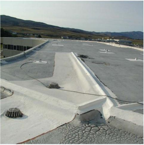
Complex drain and expansion joint configuration after 4 years of service.
