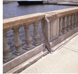
Common crack in the top rail of the balustrade attributed to expansion and contraction.
