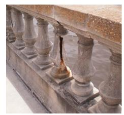
Damaged baluster revealing reinforced steel.
