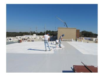
**Sika® Reemat -** a glass fiber matt embedded into Sikalatic® roof coatings for enhanced multi-directional tensile strength. Great for complex details, joints, corners, and protrusions.
