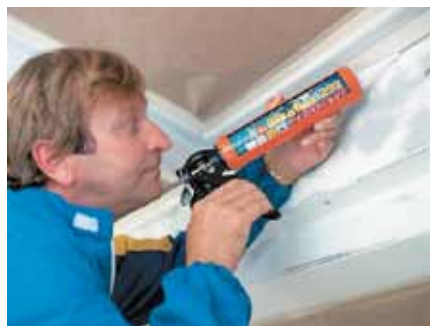
Fig. 88 Applying Sikaflex®-292
