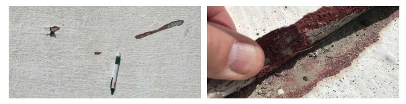
Hurricane force winds produced no peeling or delamination of the RoofPro membrane - only some skid marks and scrapes in RoofPro membrane from airborne HVAC equipment which can be easily repaired. The RoofPro membrane is still well-bonded all around the tear preventing water from getting under the membrane and moving laterally to find a leakage pathway into the building.
