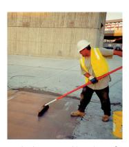
3. The longer working time of SikaQuick 1000 makes this product more conducive to larger areas of placement. Final broom finish provides for a slightly roughened surface and skid-resistance that is desirable on parking decks.
