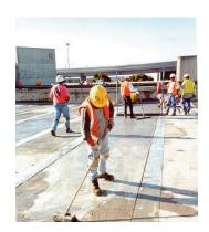
1. Scrub coat of SikaQuick 1000 is completed just prior to the placement of the overlay. This step is always required in concrete repair to ensure excellent adhesion to the existing substrate.
