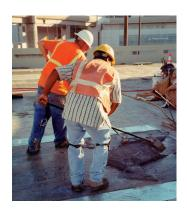
2. SikaQuick 1000 poured into place and mechanically screeded.
