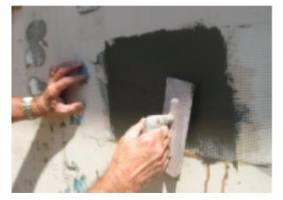
**4.** For base coats it is recommended to allow 48 hours cure time; for Finestop products 24 hours of dry time is recommended prior to pull testing. See photo.
