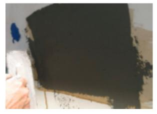
3. For the base coat, embed a 4" wide strip of Standard 4 reinforcing mesh into wet material; for Finestop products embed 4" SikaWall Sheathing Fabric into the wet material. Additional base coat or a Finestop air barrier can be applied to ensure full embedment. Use sufficient mesh or Sheathing Fabric so that 6" is embedded and 6" is left exposed for a pull tab.
