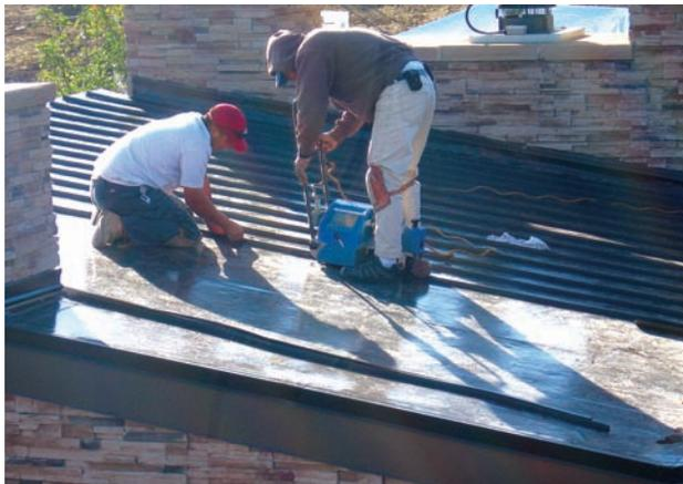
A Sarnamatic hot-air welder fuses the Décor Profile "ribs" to the membrane. Ribs are produced from the same material as the membrane, ensuring consistency of color.
