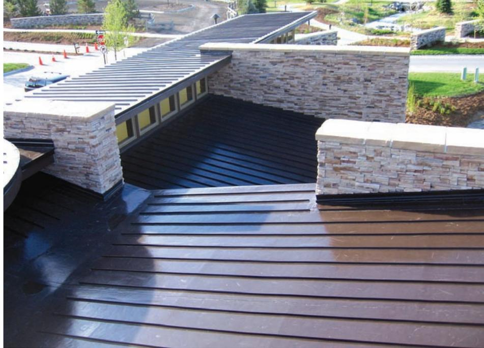
Multi-levels of the Décor Roof System, in a custom-colored bronze, handsomely finish off the Discovery Center at BackCountry. The Décor Profiles, and the larger Battens used in other Décor installations, give a roof the look of standing-seam metal.
