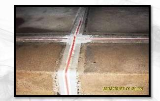
Photo: Sikadur 31, Hi-Mod Gel used as the adhesive component in the Sikadur Combiflex (SG) strip and seal expansion joint system.
