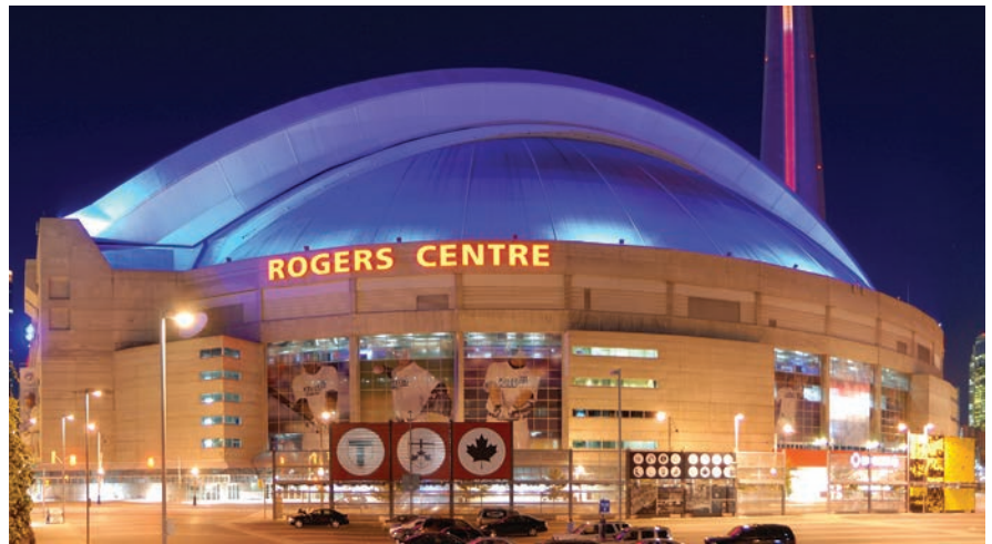
Figure 5: The Rogers Centre in Toronto, aka Skydome, was constructed in the mid-1980s and relied on 350,000 sq. ft. of thermoplastic PVC “cool roof” still in place today.
