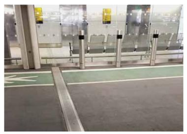
${\sf Sikafloor} {\tt @ and Sika @ Emseal movement joints working together as a complete system}.$
