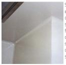
Sikagard wall systems eliminate non-sterile crevices providing seamless, rounded floor, wall and ceiling connections ideally suited for environments demanding sterile surfaces.
