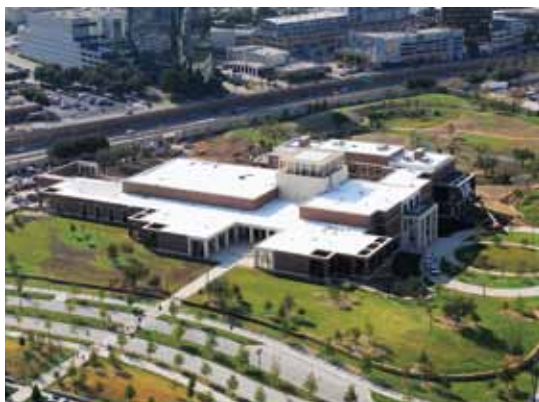
Lawrence Berkeley National Laboratory estimates that the use of cool roofing materials on 80 percent of U.S. commercial buildings would result in 10,400 GWh of cooling energy savings, and approximately $735 million in overall energy savings. Photo courtesy of Sika Corporation.
