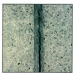
preventing water leaking through several of the joints using a silicone sealant directly over the failed joint had offered only a temporary waterproofing solution and looked aesthetically unpleasant.
