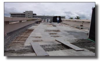
out and repeated saw cuts were made to maintain the groves. This was necessary to provide skid resistance on a 15% slope for the buses operating during Hawaii's tropical rain showers.
