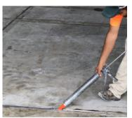
**EASY TO APPLY** With a bulk gun or plural component pump and a static mixing nozzle.
