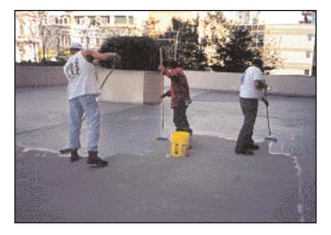
cement in the EpoCem 81 allowed the contractor to use a self-leveling mortar to temporarily stop the MVT. Once the MVT was stopped with the EpoCem, installation of the Sikafloor Traffic System proceeded.
