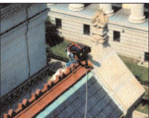
into the interior of the building. The leaks continued due to careless and spotty sealing with ineffective materials. When the decision to restore the building was finally made, it was important the building would be leak free. Because the building was very important to the City of Albany, aesthetics were also a concern. Plus the amount of joint sealing that would be required meant that the product chosen to seal all the joints would be very visible.
