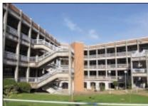
Floyd Hall Science Building is located on the Campus of North Alabama in Florence, Alabama. It is a four story concrete building with a brick and stone façade built in 1964. The building has three floors of concrete balconies each approximately 10' wide and 335' long, for a total balcony area of over 10,000 sf. The 4-inch concrete slabs were originally poured with concrete and the reinforcement placed too close to the surface resulting in insufficient concrete cover. Thirty-eight years of
