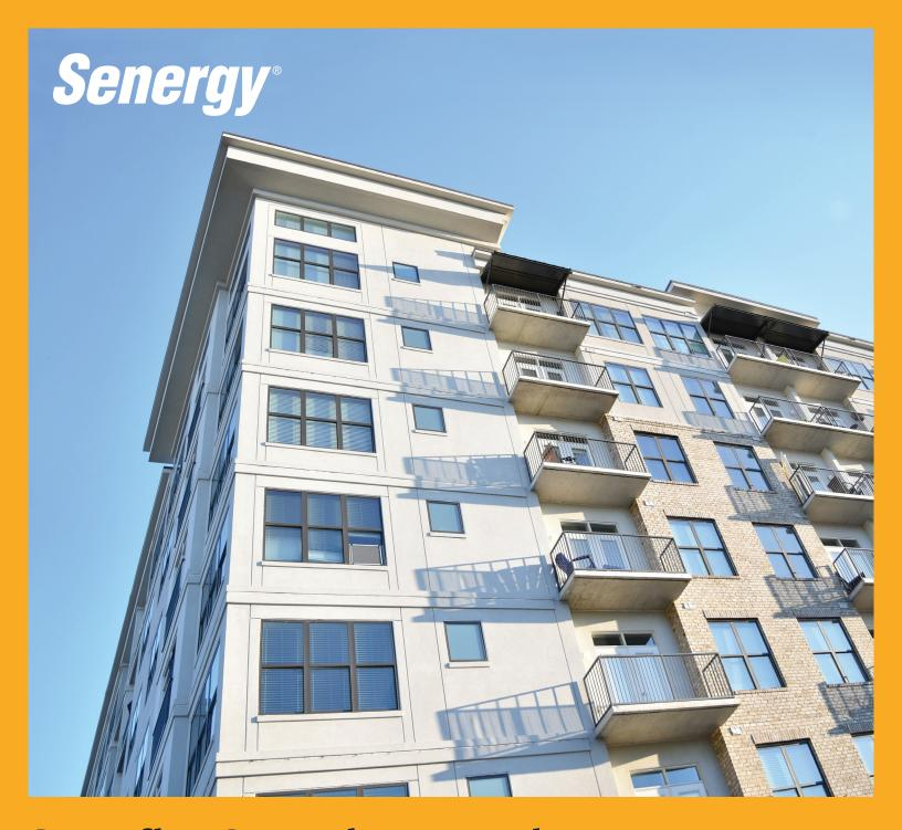
Non-drainage Class PB EIFS with Senergy Senershield air/water-resistive barrier which provides primary barrier moisture control
