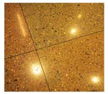
The **Class** of your SCOFIELD<sup>®</sup> Formula One<sup>™</sup> polished concrete floor refers to the level of polish that is performed on the floor. The higher the level of polish, the more glossy or shiny the floor will appear. Generally speaking, the higher the gloss, the more expensive the process will be.
